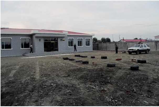
The new building for the dog handlers in Tumen and the bags set out for the dogs to train.
