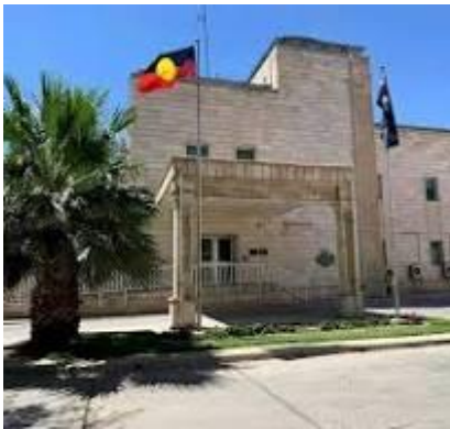
The completed Embassy
